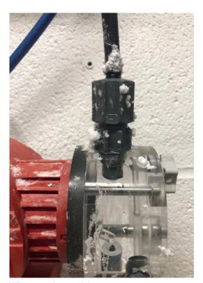
White mounds around the discharge valve of the chemical pump can be a sign of a clog within the chlorine injector.
